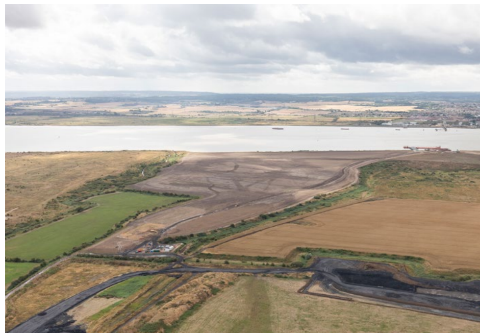
Aerial view south towards River Thames
