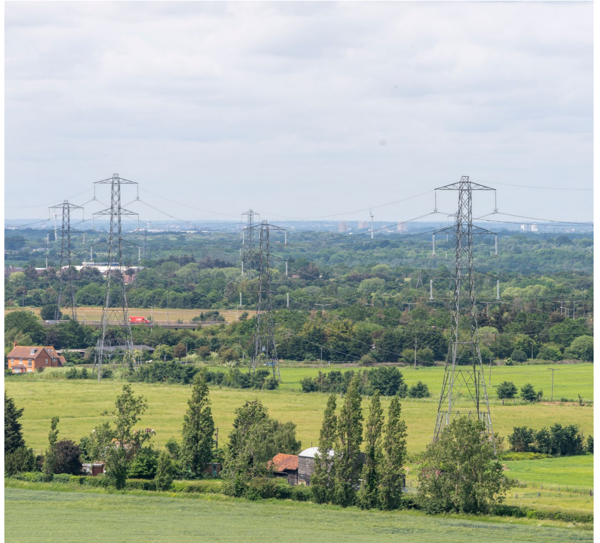
Existing pylons in the landscape. A view from Chadwell St Mary (the rooftop of Gooderham House, approximately 33m high) looking down towards the A13 Junction
