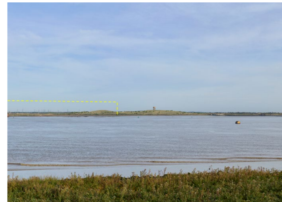
Illustrative view looking towards Tilbury Fields showing an indicative line at 50m for Tilbury Freeport
