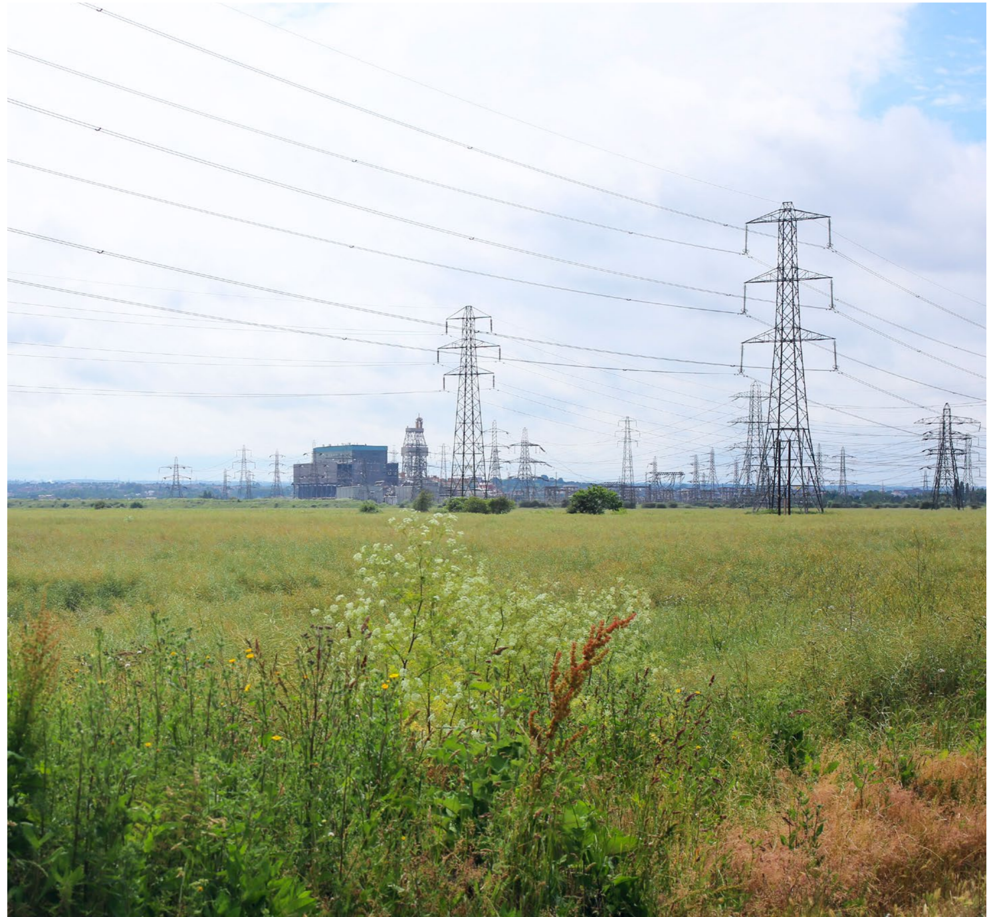
Existing pylons in the landscape at Tilbury Marshes
