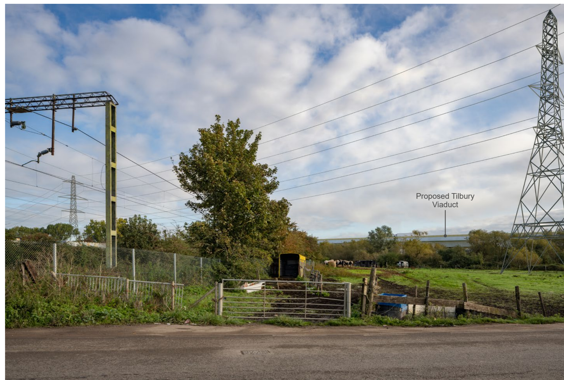
Illustrative view of Tilbury Viaduct (behind hedgerow) and utility diversions from Station Road
