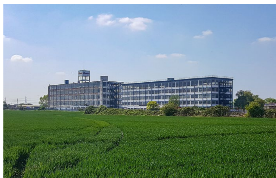
One of the Grade II listed British Bata Shoe Company factory buildings
