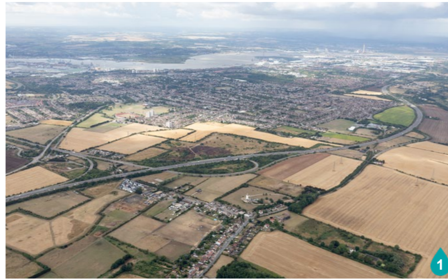
Aerial view south-west over the A13 Junction
